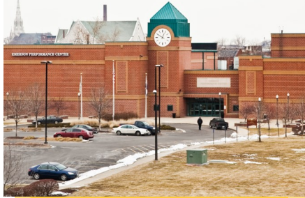
Emerson Performance Center (EPC)
